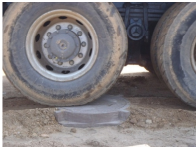
Water Cart Fourth Pass
