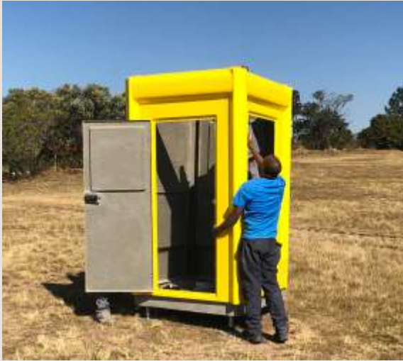
Attach right side wall to Double Sided Mullion with 5 x M6 x 20mm machine screws either side
