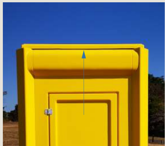
Air circulation and ventilation is provided with a 20mm gap between the top of all walls and the roof
