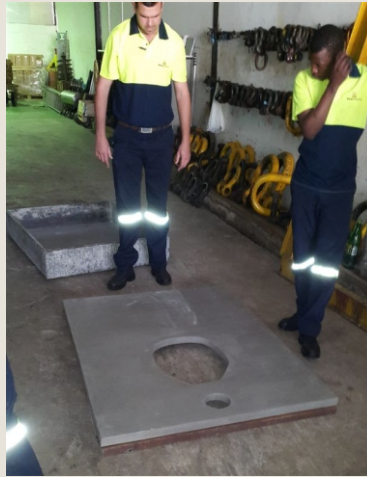
SLAB PLACED OVER "PIT LINER"
