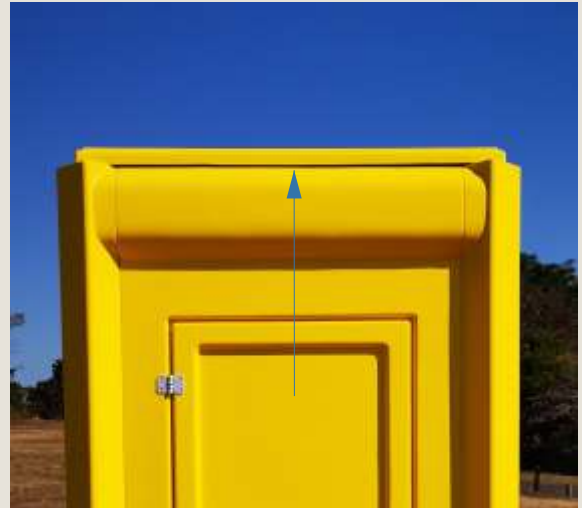
Air circulation and ventilation is provided with a 20mm gap between the top of all walls and the roof
