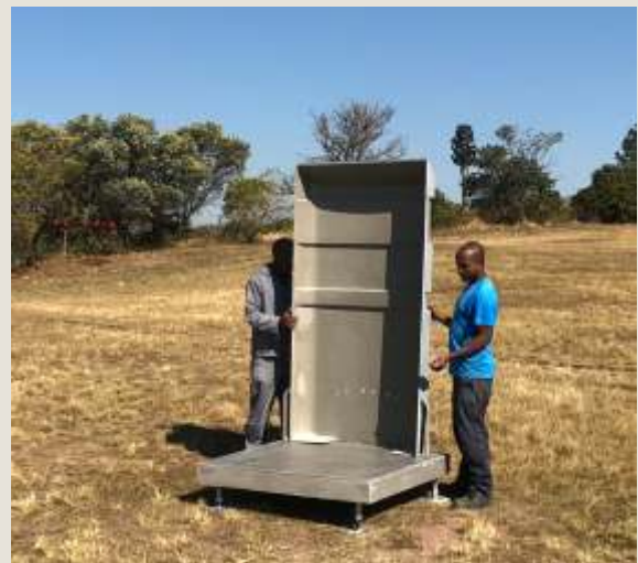
Locate the Curved Back Wall into place, by fixing down to the base with 2 x M6 x 40mm machine screws provided.
