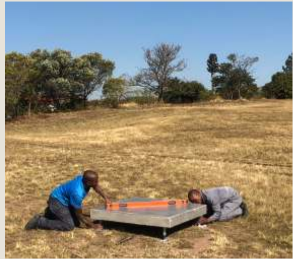
If using a StructaBond base, set the base level using the Telescopic Leveling legs
