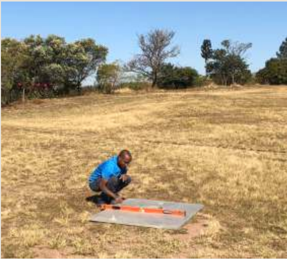
If using the structure for a VIP Pit Latrine, align the Lightweight VIP Base over the pit, ensuring that the base is straight and level
