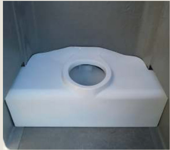
Once located, align the toilet module with the back wall and bolt into place using 6 x M6 x 20mm machine screws provided
