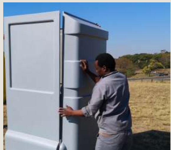
Fix the side walls into the back wall by lining up the tongue-and-groove provided and press firmly into place, wiping away any residue from the joint
