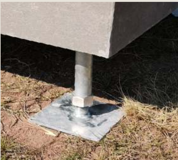
Adjust the height of the Telescopic Levelling Legs by turning the nut clock ways to go down and anti-clockways to go up
