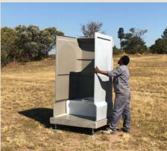
After fixing the toilet module into place, fix the side walls down to the slab using 2 x M6 x 40mm machine screws provided.
