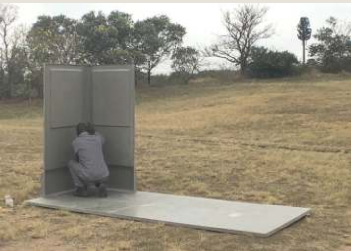
Attach the first Back Wall to the Left Side Wall using 5 x M6 x 20mm machine screws provided and then fix Back Wall down to the slab structure with suitable fixings ensuring that walls are 90 degrees to one another.
