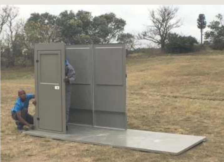
Fix the first Front Door-Wall to the Left Side Wall using 5 x M6 x 20mm machine screws provided and then fix down to the slab structure with suitable fixings ensuring that walls are 90 degrees to one another.
