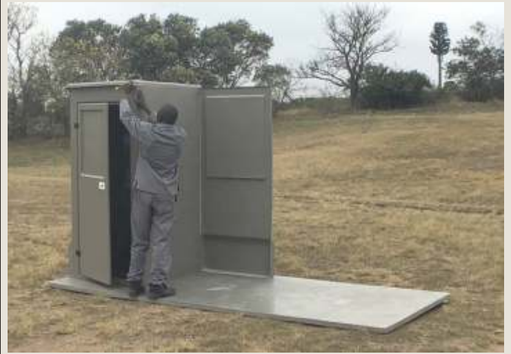
Apply a bead of Structural Polyurethane along the top of the Side wall and install the Left Side Roof into place, aligning the right hand side flange of the Roof into the top of the Mid Wall and locking the Roof into place over the Back and Door-Wall.
