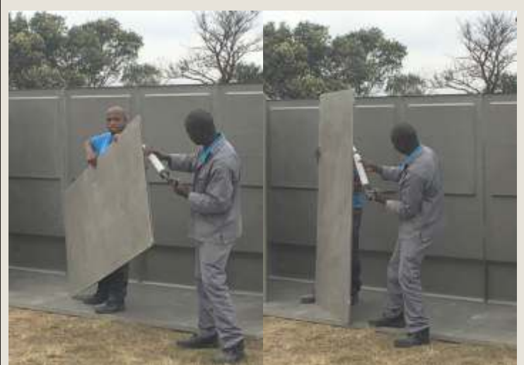
Apply a full bead of Structural Polyurethane into the groove along the entire length of both sides and the top of the first Mid Wall, ensuring that there are no gaps - this is critical to ensure that there are no leakages.
