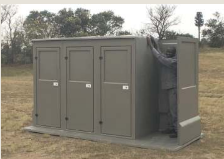
Install the next Mid Roof into place, aligning the left and right hand flanges into the top of the Mid Walls and locking the Roof into place over the Back and Front Door-Walls.
