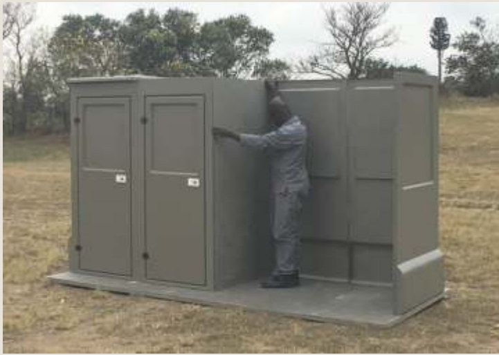
As with the first Mid Wall, apply a full bead of Structural Polyurethane into the groove along the entire length of both sides and the top of the next Mid Wall and install into place aligning flanges of the Back Walls and Front Door-Wall into the groove of the Mid Wall wiping away excess Structural
