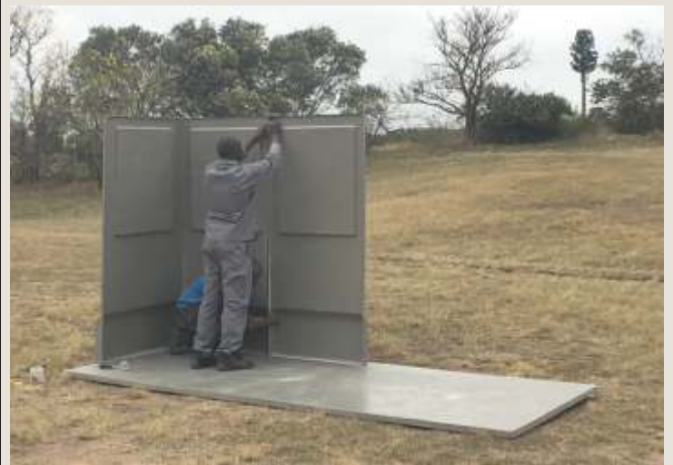
Locate the second Back Wall into place, and attach to the First Back wall with 3 x M6 x 20mm machine screws provided, then fix to the slab structure with suitable fixings.
