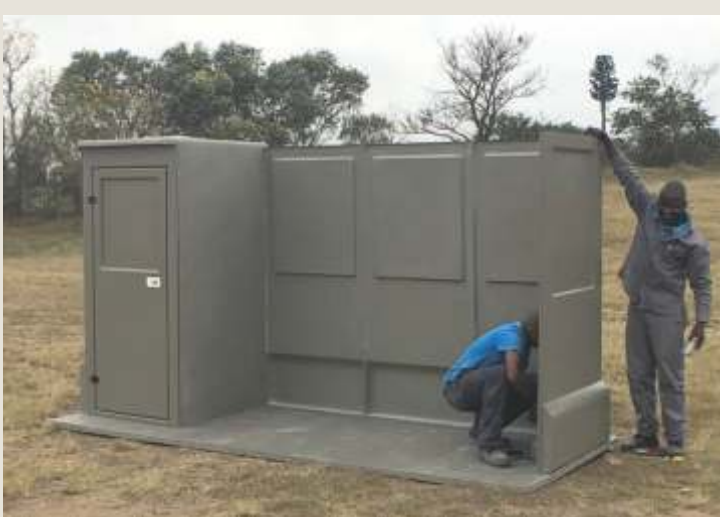
Fix the Right Side Wall to the last Back Wall using 5 x M6 x 20mm machine screws provided and then fix down to the slab structure with suitable fixings ensuring that walls are 90 degrees to one another.
