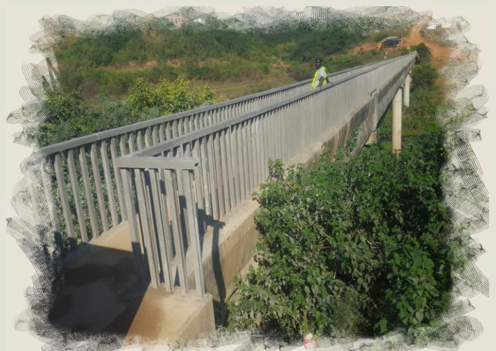
Pedestrian Bridge WS3 - Umlazi
