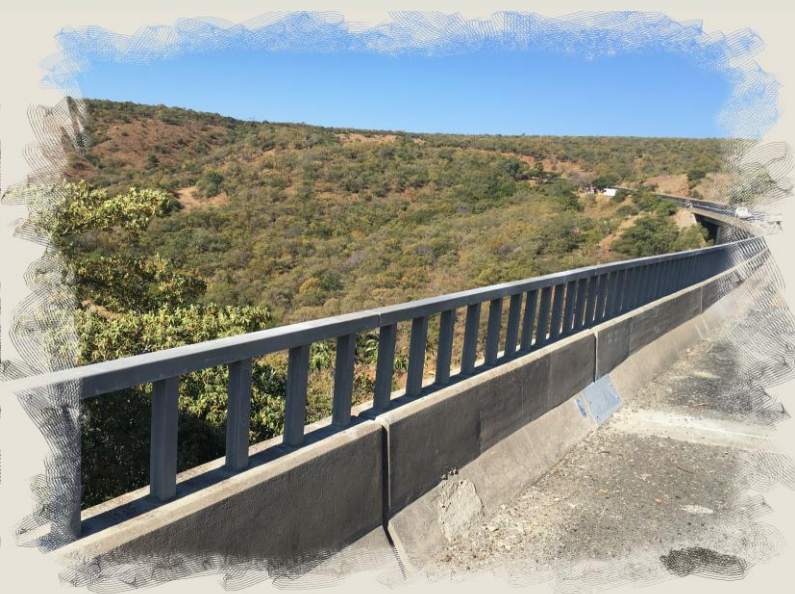
Concrete Barrier Parapet Handrail - Ulundi
