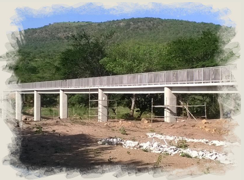
Pedestrian Bridge - KwaMbonambi
