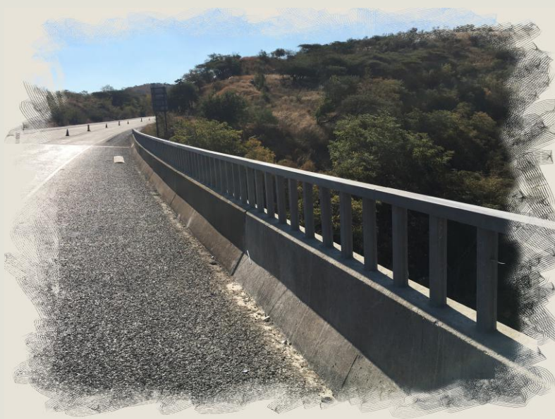
Concrete Barrier Parapet Handrail - Ulundi
