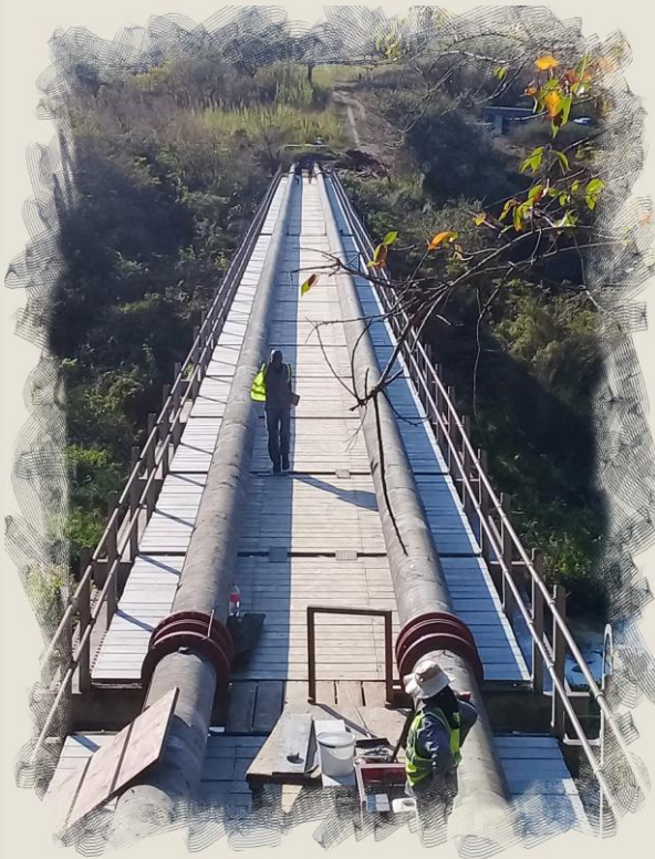
Pipe Bridge 73 Handrails & Decking - Umlazi
