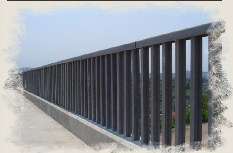
Pedestrian Bridge M1 - Shallcross Durban
