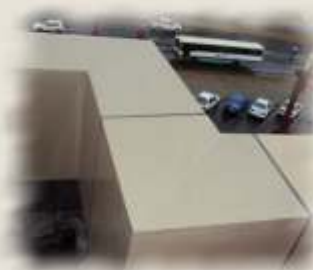
MODUBOND ON STAINLESS STEEL TOP-HAT BRACKETRY SYSTEM INCORPORATING 3M VHB ADHESIVE TAPE
